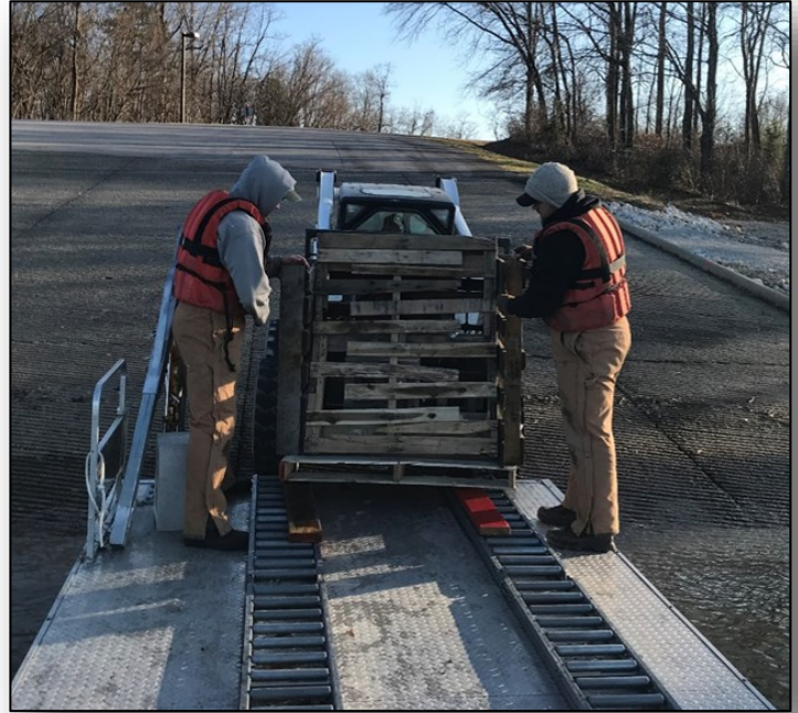
Loading structure onto pontoon boat. Sam Peterson and Craig Jansen from the Big Rivers crew load up a structure being delivered by Wayne Meyers in the skidsteer (Sugar Ridge laborer).
